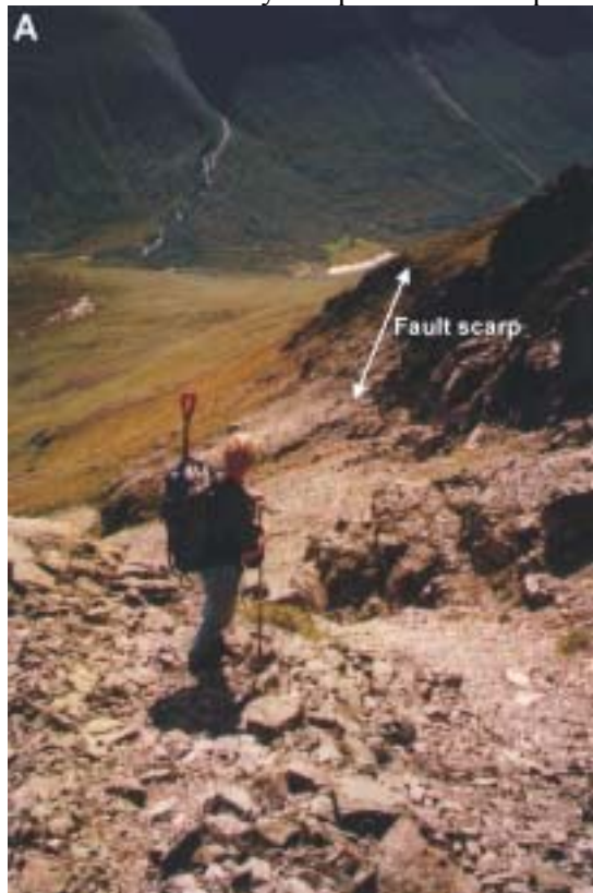
Figure 40. The Berill fault is well exposed in bedrock high on the mountain slope. The fault scarp is unstable, as documented by minor rock falls.
